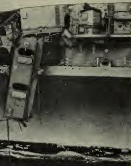
GREEN SEA broke over Valley's deck ripping loose an area 70 feet long from the carrier's port side.
